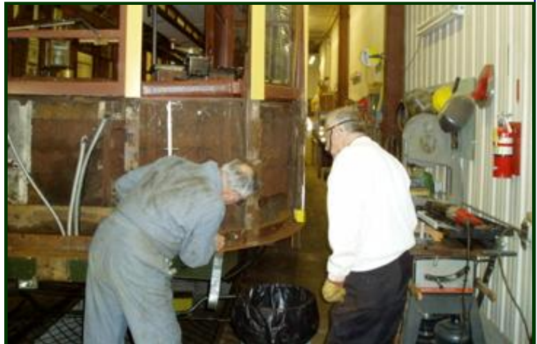
Progress on No. 1300. Tom Fairbairn (left) and Russ Isbrandt have been part of the crew making good progress on the front end work of No. 1300. (Jim Vaitkunas photo)
