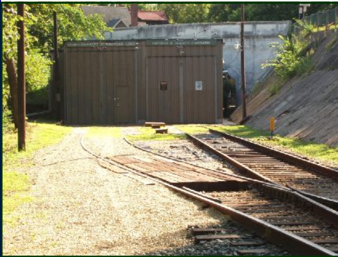
This photo shows the new “crossing” over the Isaacs car barn maintenance barn lead track. Now delivery trucks and automobiles can cross over the rails and snuggle right up to the car barn door without tearing up a tire or two. ( John Prestholdt photo )
