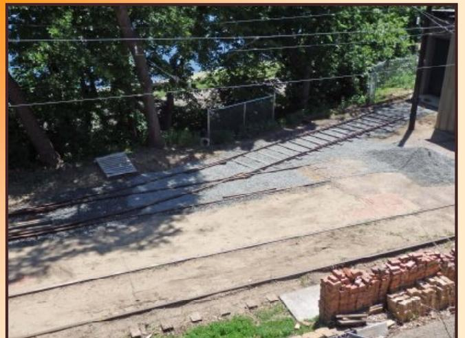
On June 6, 2017 good progress was made building the track into the speeder shed. Ballast stone was put down and spread and initially tamped. Soon the short curved track will be built up to the speeder shed door and the switch stand will be installed. *(Dennis Stephens photo)*
