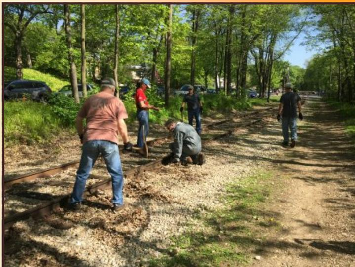
Maintaining the track is an important task at the Museum. Here we see the crew working on tightening track bolts and pounding down loose spikes. *(Keith Anderson photo)*
