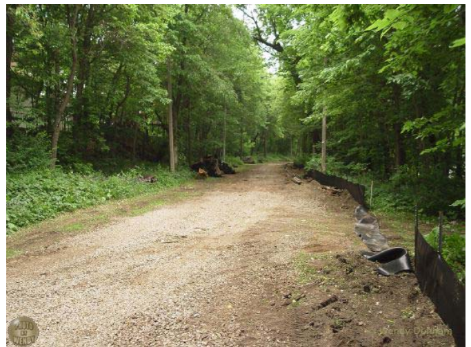
(Top) Cottage City and the "S-curve" after the track was lifted (6-3-05).
