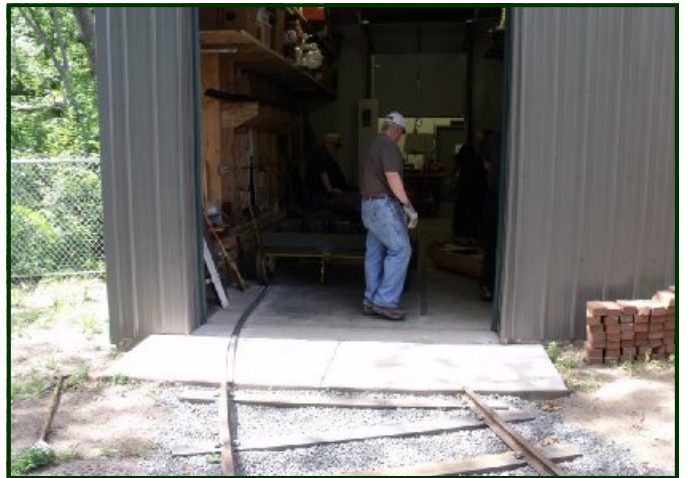
(Left) Ben Franske, John Prestholdt and Jim Willmore testing the new track with a work flatcar. (Above) The track into the shed isn't regular T-rail, but steel shapes, with the work cars rolling on their flanges. (Jim V photo)
