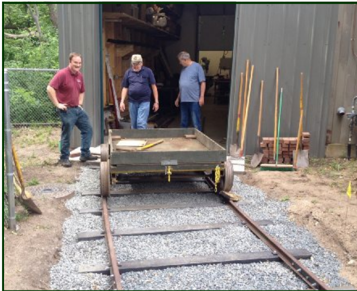
Jack Bacon looks happy using the rail bender. We used steel ties to support the rails (25 pounds-per-linear-yard) and maintain the correct track gauge, rather than the usual wood ties.
