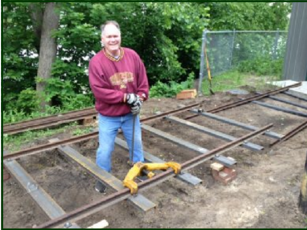
Jack Bacon looks happy using the rail bender. We used steel ties to support the rails (25 pounds-per-linear-yard) and maintain the correct track gauge, rather than the usual wood ties.
