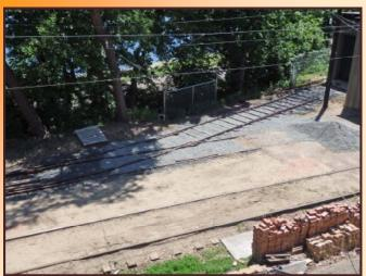
On June 6, 2017 good progress was made building the track into the speeder shed. Ballast stone was put down and spread and initially tamped. Soon the short curved track will be built up to the speeder shed door and the switch stand will be installed.
