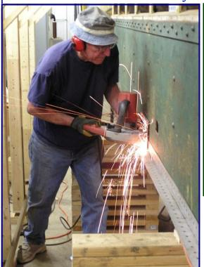
(Left) Ken Albrecht is using the special steel-cutting saw to cut through the steel side of Winona No. 10. The metal angle on the bottom is being used as a guide to keep the cut straight.
