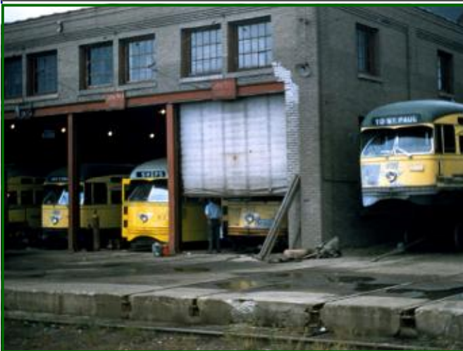
TCRT's Snelling Shops was a complete shop. These two photos show several TCRT PCC cars in the process of being modified for their service on the Shaker Heights Rapid Transit line in Cleveland, Ohio. All the work to repair the cars, paint and letter them and install the multiple unit controls that SHRT wanted was accomplished by the Snelling Shops artisans. (MSM Photo Archive)
