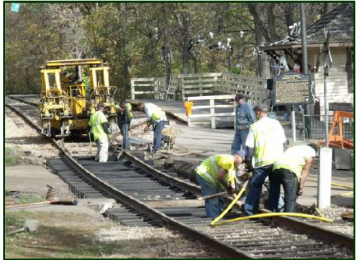
(Top Left) By the time your photographer arrived on the scene on October 19 th , the trench was cleaned out, the new ties were put in and the two pieces of welded rail were placed on the ties and tie plates. Note the pile of trap rock ballast stone on the right. (Top Right) Spiking the track to gauge has now begun. The implement in red is a pneumatic spike driver. (Bottom Left) Some things still have to be done the old fashioned way. Note the welded joint opposite the Rail Specialties worker. (Bottom Right) Two crews are working at each end of the crossing. The trackwork was finished in two days. In the rear is the tie tamping machine that will raise and level the new track. The City of Minneapolis was responsible for the asphalt work which happened the day after.
