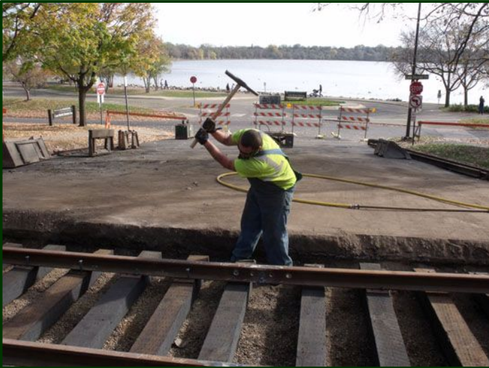
(Top Left) By the time your photographer arrived on the scene on October 19 th , the trench was cleaned out, the new ties were put in and the two pieces of welded rail were placed on the ties and tie plates. Note the pile of trap rock ballast stone on the right. (Top Right) Spiking the track to gauge has now begun. The implement in red is a pneumatic spike driver. (Bottom Left) Some things still have to be done the old fashioned way. Note the welded joint opposite the Rail Specialties worker. (Bottom Right) Two crews are working at each end of the crossing. The trackwork was finished in two days. In the rear is the tie tamping machine that will raise and level the new track. The City of Minneapolis was responsible for the asphalt work which happened the day after.
