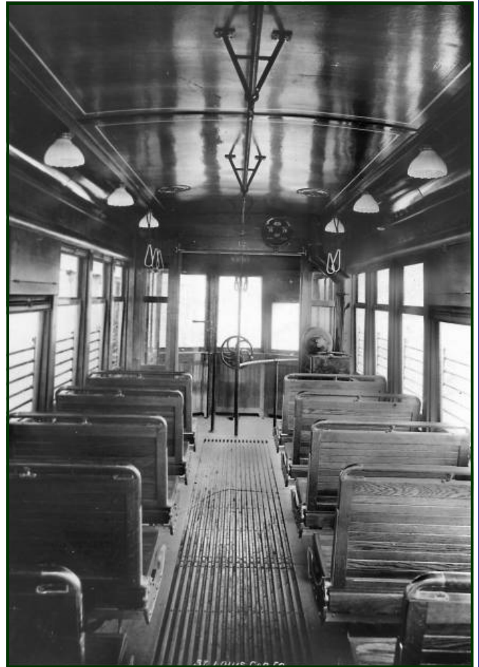
Above Right. This photo shows the interior of Winona No. 12, sister car to our No. 10. This is the official St. Louis Car Company photo taken just prior to shipping the car to Winona. The cars (Numbers 9 to 12) were delivered in 1914. We will restore the interior of No. 10 car as shown in this photo. (MSM Archive Photo)
