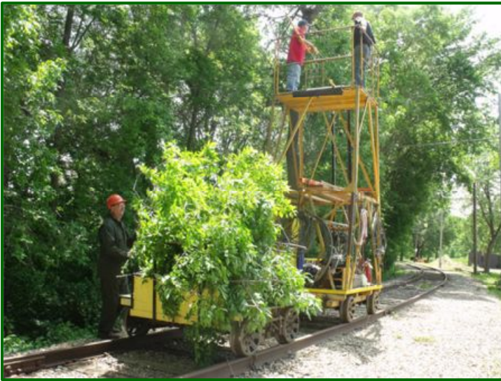
That's Dave French on the ground assisting Rod Eaton and Bill Arends on the tower wagon. The initial task for the morning's work was to re-paint all of the overhead targets on CHSL and to re-position a couple of them. But along the way a lot of limbs were near to or touching the overhead trolley wire, and the crew had to take care of that problem. These two photos show the crew in the archery range curve area of our Como-Harriet Streetcar Line. ( Jim Vaitkunas photos )
