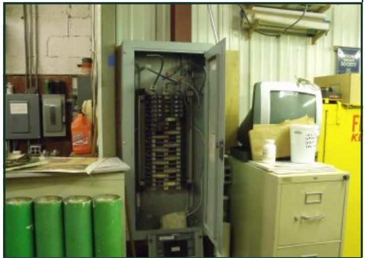
Major electrical work needs to be done before we can build the bathroom in the Isaacs carbarn. Here's a photo of the new main shop panel. To the left you can see electrical panels and disconnects mentioned above that'll have to be removed to make way for the bathroom.
