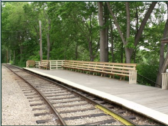
New benches at Linden Hills. The fellows took off a Tuesday from normal shop and restoration work and replaced the old benches at the Linden Hills station. They look real good. (Photo by Jim Vaitkunas)
