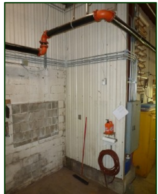
Before and After Photos. As you can see, the corner is now cleaned out and ready for the next phase of our George Isaacs carbarn improvements project. Next step: the sewer line needs to be installed. Then the plumbing for the toilet and sinks can be finished. Our shop volunteers will most likely frame-in the bathroom itself. The large black pipe above where the bathroom will go is part of the sprinkler system. The new electrical panel mentioned in the article can be seen on the lower right of the photo. (Dennis Stephens photos)
