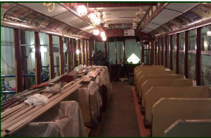
(Above) No. 265's interior is a mess at the moment. Rattan seat cushions and backs are being refurbished and painted. Why are we painting the seats the buff color? Because that's what TCRT and DSR did starting in the 1920s to prevent lady's silk stockings from being snagged by small fibers from the rattan. (Jim Vaitkunas photo)
