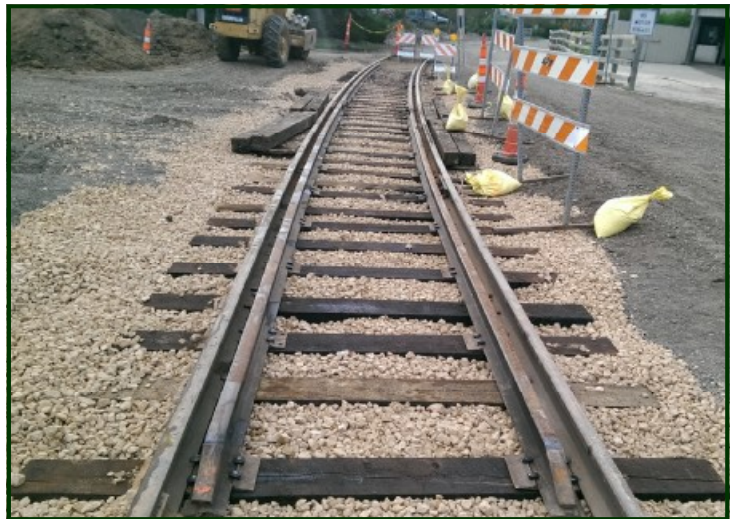
At ESL, the sewer work on Morse Avenue is mostly done and our track is back in place. Next step: paving the street. (Todd Bender photo)
