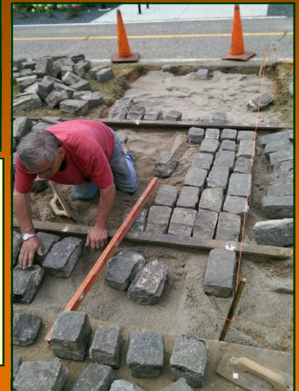
(Above) MSM member Bob Woodburn and Excelsior historian Bob Bolles have marked where the TCRT pavers will go. Next step is to dig out the grass, put down a bed of construction sand and lay the pavers.
