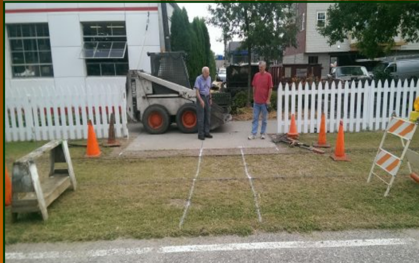
(Above) MSM member Bob Woodburn and Excelsior historian Bob Bolles have marked where the TCRT pavers will go. Next step is to dig out the grass, put down a bed of construction sand and lay the pavers.
