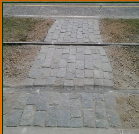
(Above) MSM member Bob Woodburn and Excelsior historian Bob Bolles have marked where the TCRT pavers will go. Next step is to dig out the grass, put down a bed of construction sand and lay the pavers.
