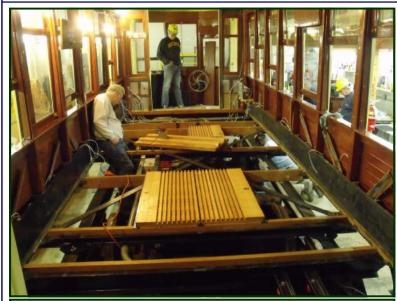
**Dick Zawacki** is shown here working on fitting the floor traps. The floor traps are removable to allow access to the motors for servicing. (*Jim Vaitkunas photo*)
