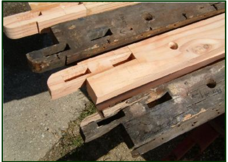
(Above) This photo shows some of the wood pieces that make up the substructure of Winona No. 10. In both instances the pieces were either broken (as you can see in the foreground) or suffered dry-rot damage making the piece, or a portion of the piece, unusable. (Photo by Ken Albrecht)
