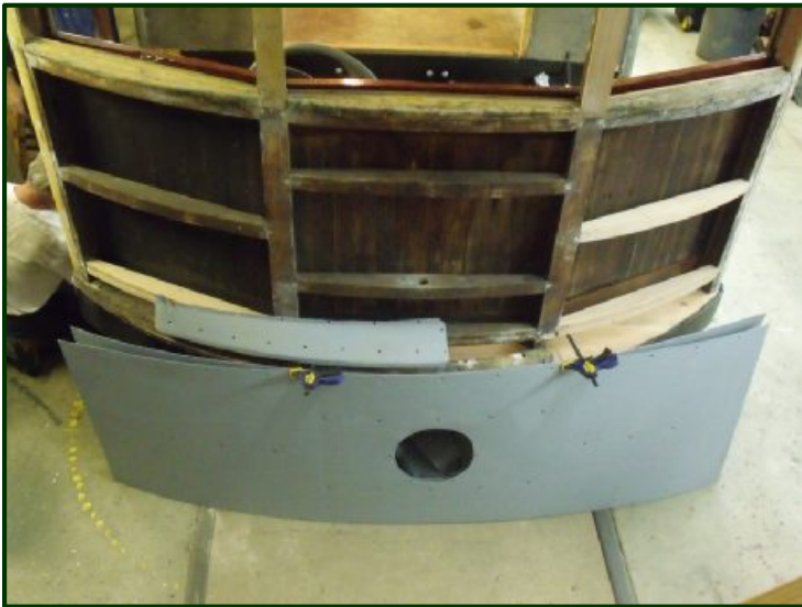
Here a close-up of the end of Winona No. 10. The metal dasher panels have been primed but are not yet ready to be installed. Note the obviously new pieces of wood. Some of the old wood pieces were rotten beyond re-use. (Jim Vaitkunas photo)
