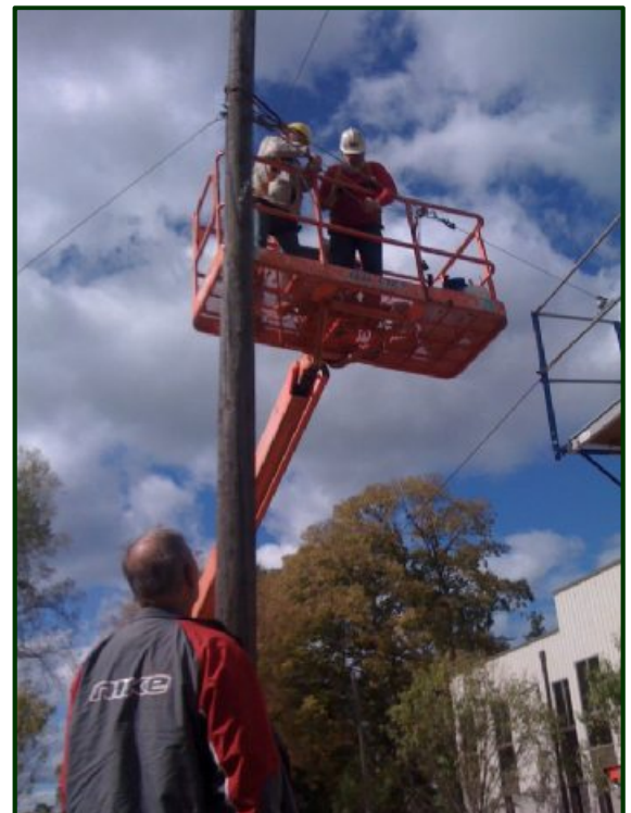
(Above) This “man-lift” machine was essential to the success of this project. As you can see from the photos in this supplement, much of the overhead work, and the tree trimming, was done away from the track in the area of the support poles. The tower wagon could not be used to work on the line poles themselves.
