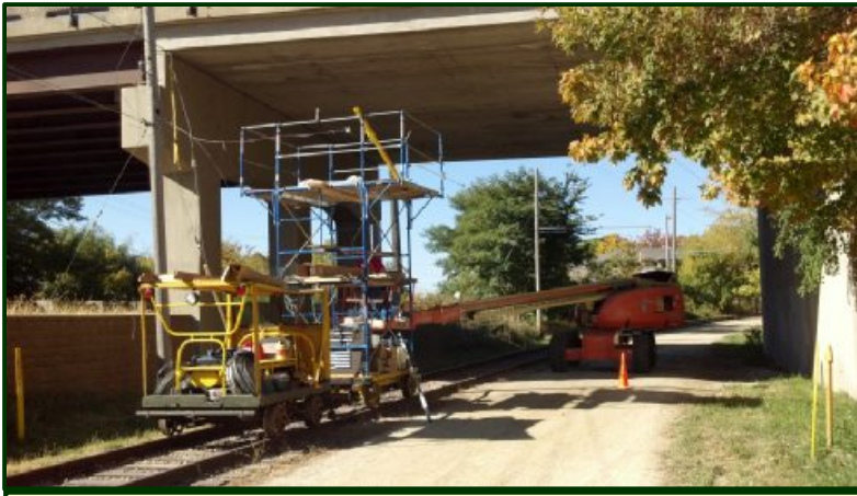
Working on the bracket arm next to the Mill Street bridge.
