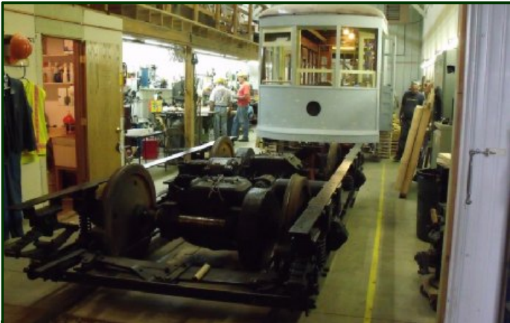
The Dupont model single truck was delivered on May 7, 2014. Soon the body of No. 10 will be jacked-up and the truck will be rolled under the car. When the body is lowered onto the truck, for the first time in 76 years, No. 10 will be sitting on powered wheels! (Jim Vaitkunas photo)
