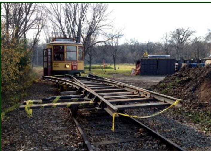
On Tuesday, November 15 th , No. 265 towed the switch to the Isaacs car barn for installation the next day.
