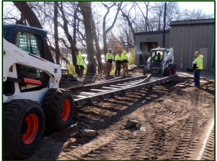
The switch is put in place by the two bobcats.
