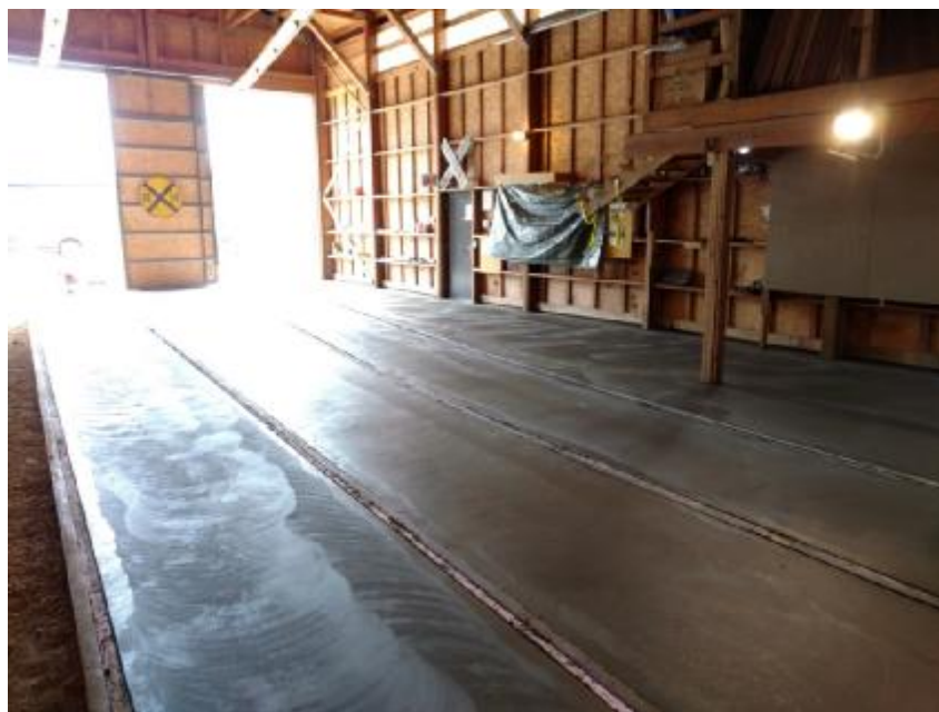
Concrete floor at ESL car barn
