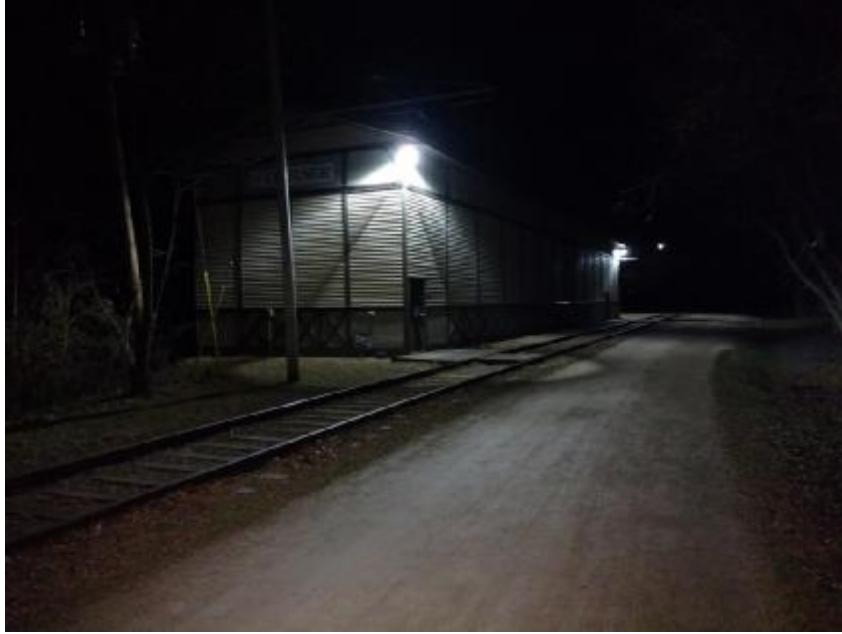
Exterior lights at ESL car barn
