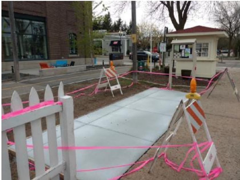
Concrete pad at Water St
