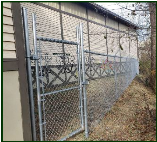
A new fence was installed on the south side of the ESL car barn to hopefully keep the taggers out. (Karen Kertzman Photo)
