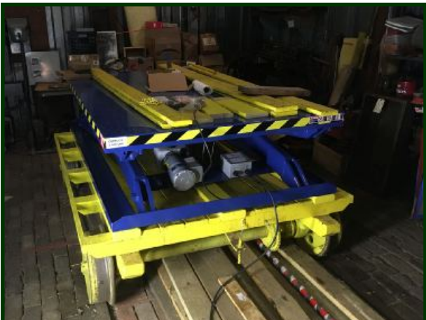
The new tower car for CHSL is being built by Dennis Stephens and some of the George Isaacs shop crew. The top six-feet of the old tower car will be placed on the scissors lift shown in this photo. (Aaron Isaacs photo)
