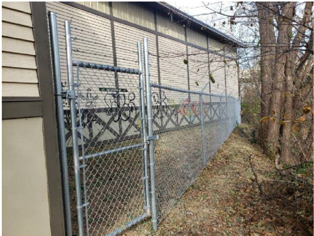
Barbed Wire Fence Installed
