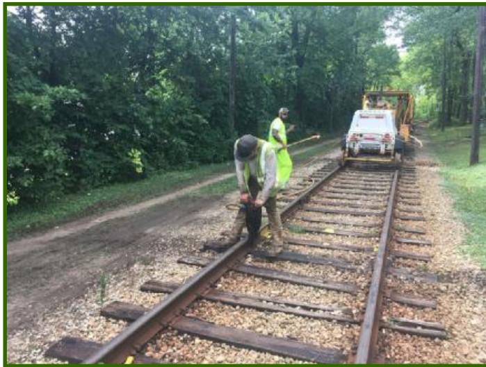
Driving new spikes into installed railroad tie. (Photo by Aaron Isaacs)
