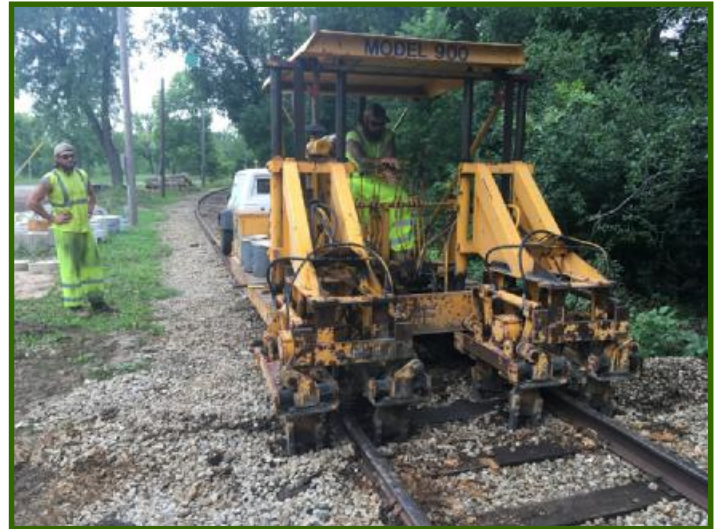
Tamper gets the ballast stone under the tie. (Photo by Aaron Isaacs)
