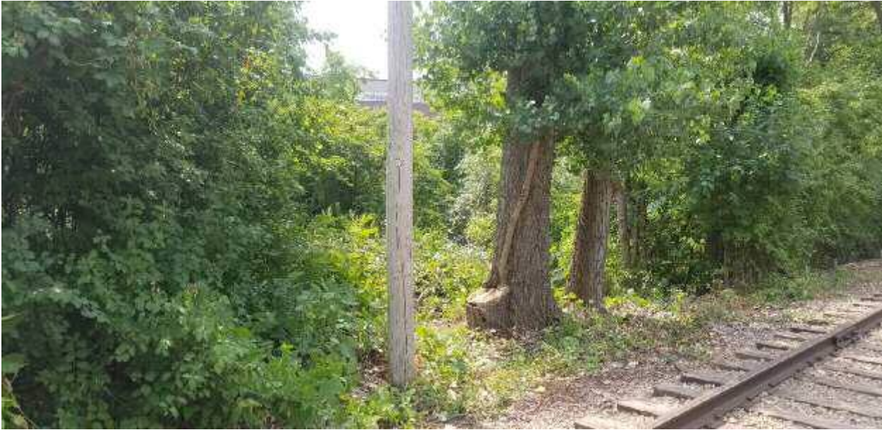
Pedestrian Path After Brush Clearing
