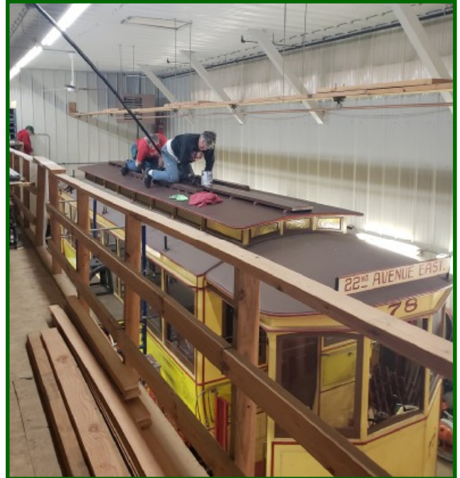
Duluth No. 78's roof is being cleaned to prepare it for repainting. Carl Floren and Jerry Draeger are on the roof, with Scott Heiderich in the background. (Jim Kertzman photo)
