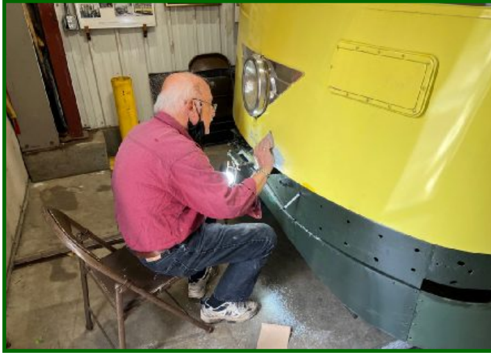
Back several years ago, a switching accident in the Isaacs carbarn resulted in damage to the front of PCC No. 322. Here we see Mike Miller doing the repair work on the car's front. (Aaron Isaacs photo)
