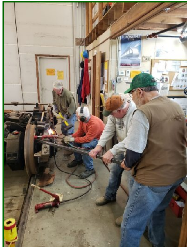
(Right) Both Baldwin trucks were built under license in Kobe Japan. During shipping to the U.S., the frames were bent. To get both trucks back to operational condition, the frames needed to be straightened. Here we see Howie Melco heating part of the truck's frame while Scott Wardrope uses a mallet to straighten it. Scott Heiderich and Dick Zawacki use a bar to apply pressure to the frame to help the process.
