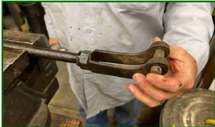
A pair of fixes to TCRT No. 1300's front doors are underway. The photo shows part of the linkage that opens the doors. Opening and closing the doors didn't feel right and here's the answer. The bushing that Tom Schramm is holding has worn its holes to a bigger diameter so it's loose. The fix is to replace the bushing with a bigger one that will fit the holes snugly.
