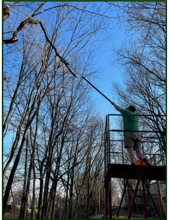
(Above Left & Above) The new CHSL tower car in action. The spring wind storms we had brought down limbs and branches onto the trolley wire. So a crew consisting of Bill Pekarna and Jerry Betz went down the line and cleared the limbs off the overhead. (Both photos by Jerry Betz)
