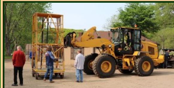
After the tower wagon was derailed and moved in the Park Board's maintenance area at Bde Maka Ska, a heavy-duty forklift was used to lift the tower wagon on to the transporting trailer.
