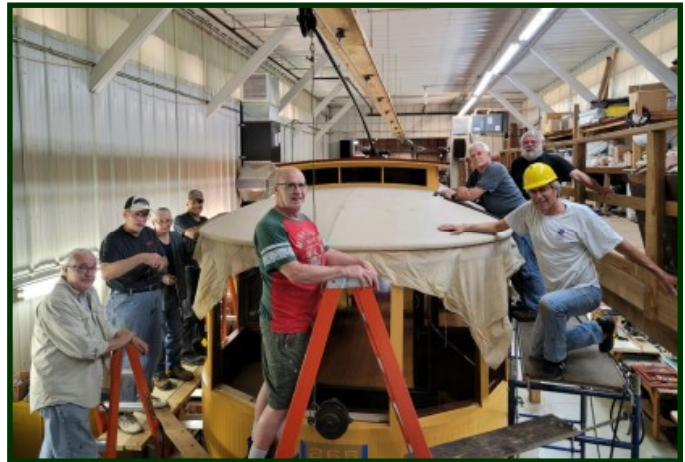
The ESL Shop Crew is shown stretching the canvas over the repaired roof on DSR No.265. From back left to right: Tom Heimer, Scott Wardrope, Jerry Draeger, Mike Kimitch, Chuck Bingham (on ladder), Carl Floren, Howie Melco, and Steve Mages . (Photo by Dave Buckman)
