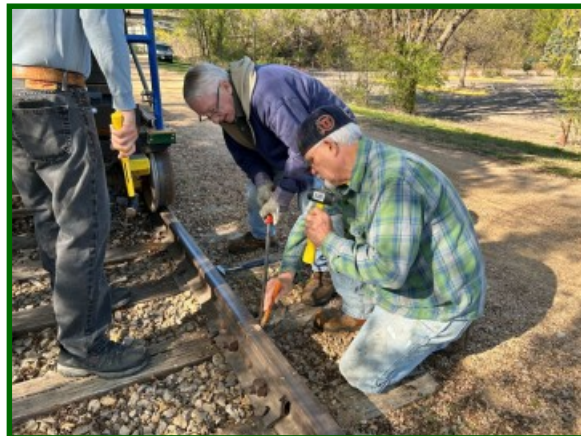
Tom Heimer, Scott Wardrope, and Howie Melco are seen here repairing a rail bond at ESL.
