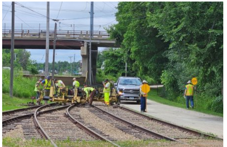
Gregg Thomas and Jerry Draeger (with yellow stop signs) monitoring the trail traffic while Railroad Specialties replaced 72 railroad cross-ties on the ESL line. (Karen Kertzman photo)
