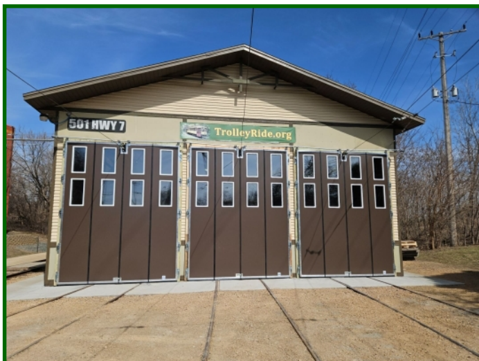
The ESL carbarn has a new set of doors! The old ones were difficult to operate and were in danger of falling off the roller track. These new ones are easier to operate, more secure and let some light into the unheated part of the carbarn. (Karen Kertzman photo)
