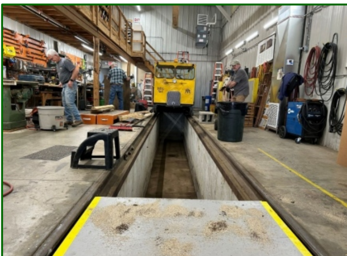
It's pit cleaning day so the pit can be ready when Mesaba 10 is pulled into the shop portion of the ESL carbarn. Pictured are Howie Melco , Tom Heimer and John McElmurry hard at work. (Karen Kertzman photo)
