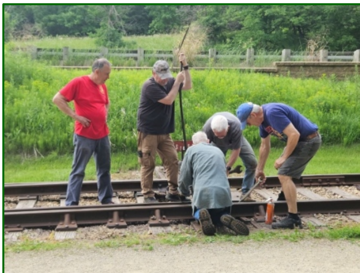
Switch alignment: Eric Werner, John McElmurry, Scott Wardrope, Howie Melco and Tom Heimer are adjusting switch points in the ESL car barn yard. (Karen Kertzman photo)
