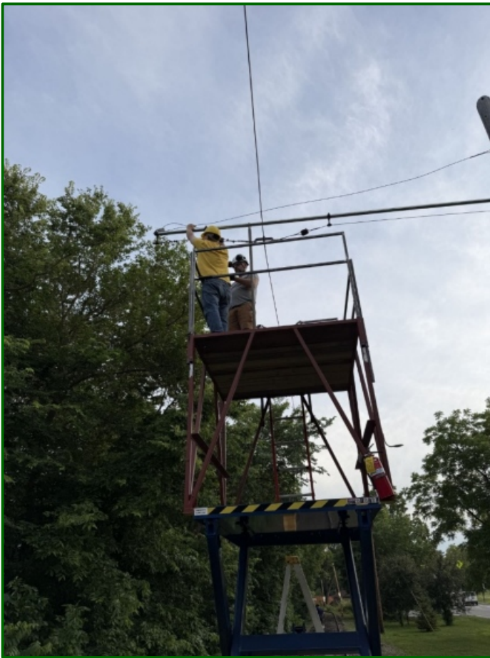
(Left) Chris Heck & Scott Brar are wrapping up installing the new bracket. (Right) A special prop was used to support the heavy bracket arm so Chris and Scott on the tower car didn't have to manually hold up the heavy bracket arm while the final work was completed. Good job guys! (Jerry Betz photos)
