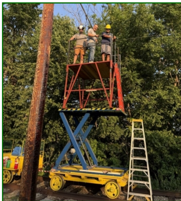
The overhead line crew replaced the second bent bracket arm. On the tower car from left are: Chris Heck , Scott Benson and Scott Brar . (Photo by Jerry Betz)
